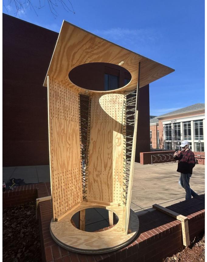
03 Assembled: perforated panels and cord strapping
